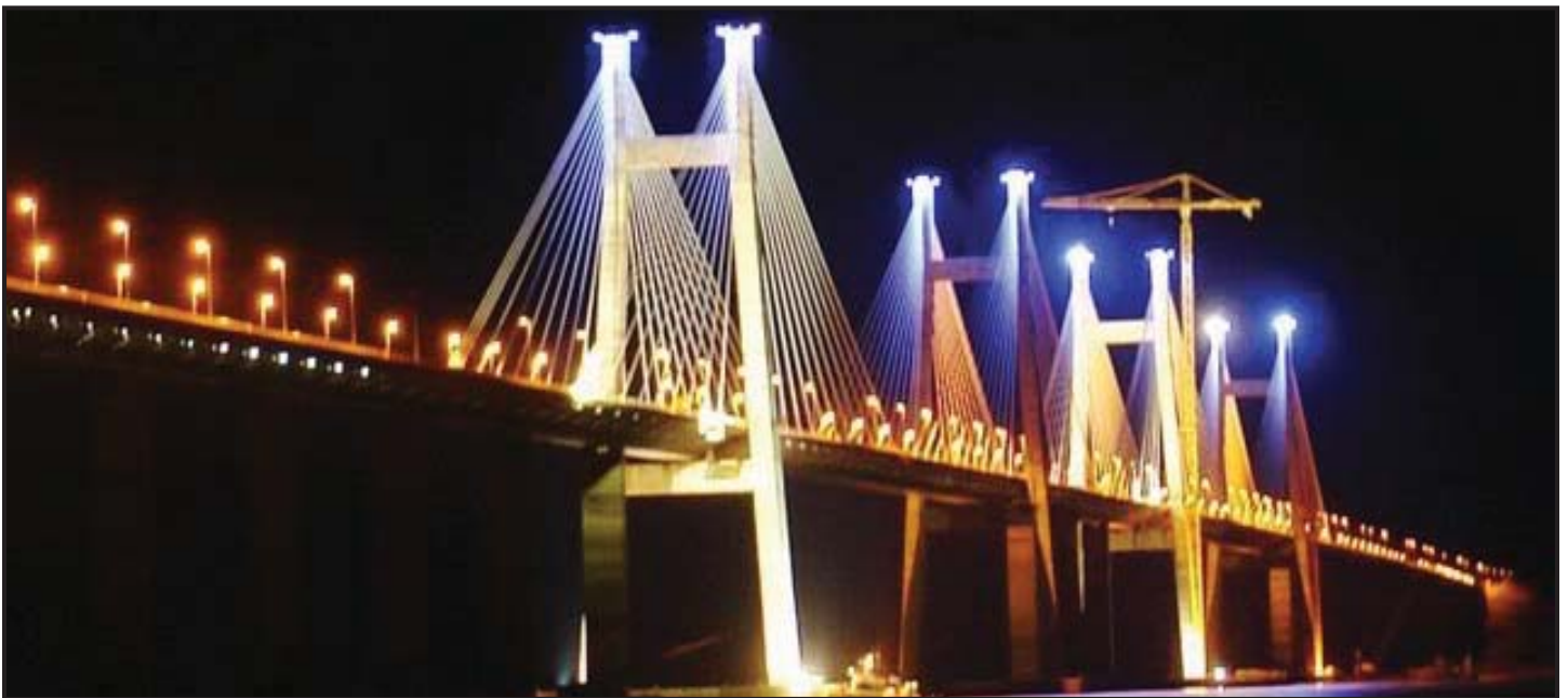
KRB equipment was used by Odebrecht to cut and bend the massive steel requirements for the Orinoco River Bridge.
